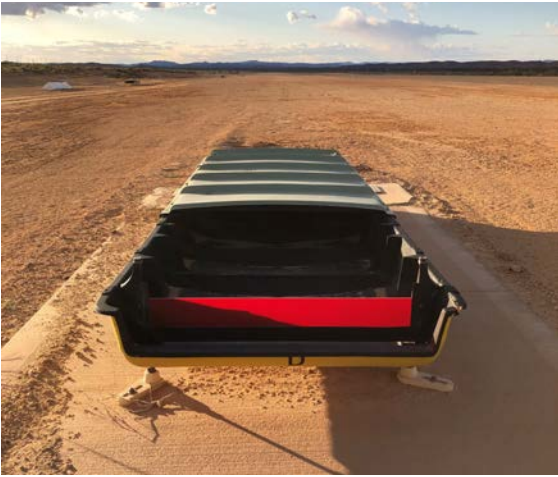
The old TVASIS (Visual Approach Slope Indicator System) and the new PAPI (Precision Approach Path Indicator)
